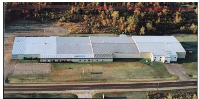
Coilmate Dickerman's 80,000 sq. ft. facility in Clinton, ME
